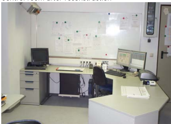
Control room after reconstruction
