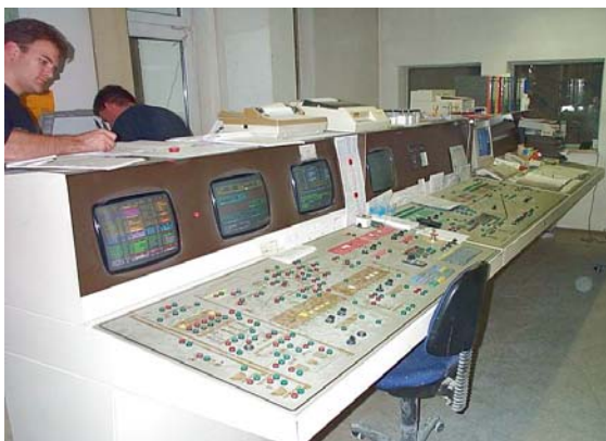
Control room before reconstruction
